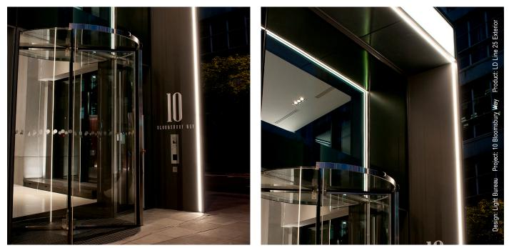
The new LD Line 25 is an exterior rated LED homogenous line of light. It is custom made to suit the dimensions on site. Cut increments of 50mm allow lengths to fit into most details, with minimal dark spots. Please note that LD Line 25 Exterior is not suitable for external applications within the floor / ground. LD Line 25 can be mounted internally into the floor / ground, but only in areas of low footfall.
